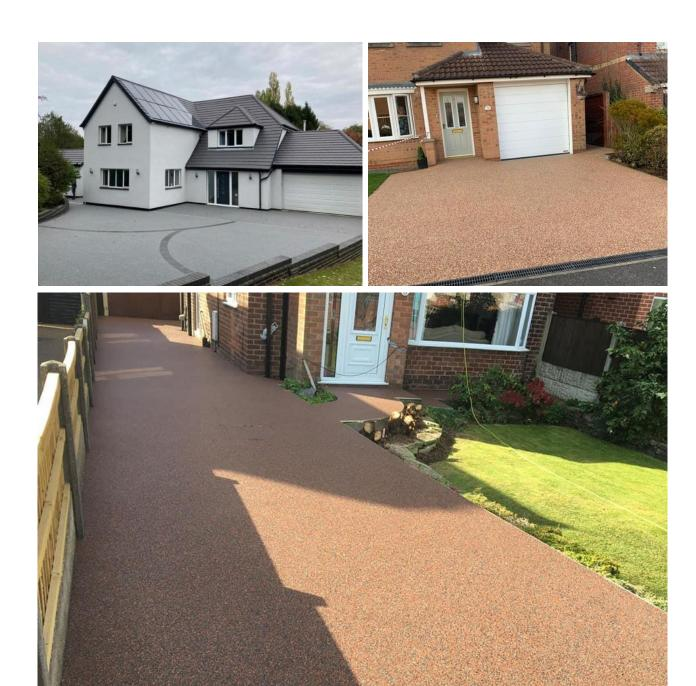
Unlike block-paving or concrete, Resin surfaces do not lose their colour over time due to sunlight exposure. To clean a Resin driveway, a simple sweep and washdown with a pressure washer is sufficient to bring it back to its former glory.
